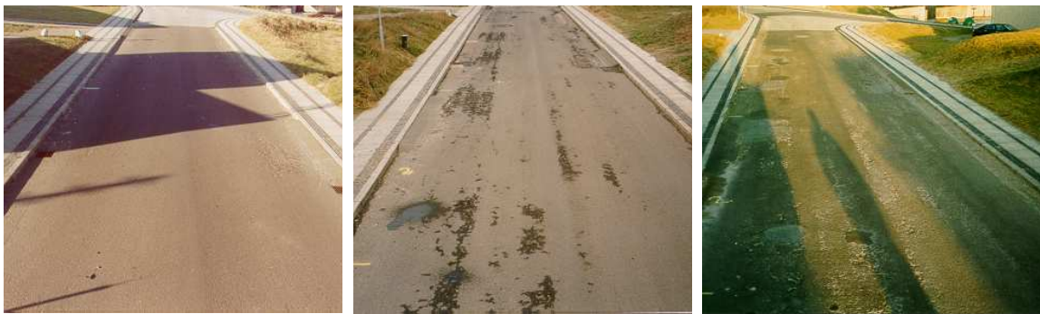
Figure 13. Example of visual condition of 10 meters of a test section in 1989, 1994 and 1999
